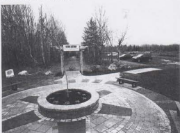
The new Rotary Gateway at the north entrance to Riverview's Mill Creek Nature Park at the end of Runnymede Road
